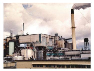
The composition of the flue gasses is typical for a kraft pulp mill and includes carbon dioxide, oxygen, sulfur dioxide, reduced sulfur, water and particulates.
